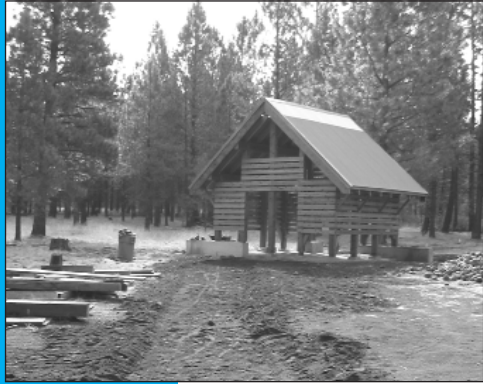
The Metolius Preserve South Fork kiosk under construction with support from the HEDCO Fdn.
