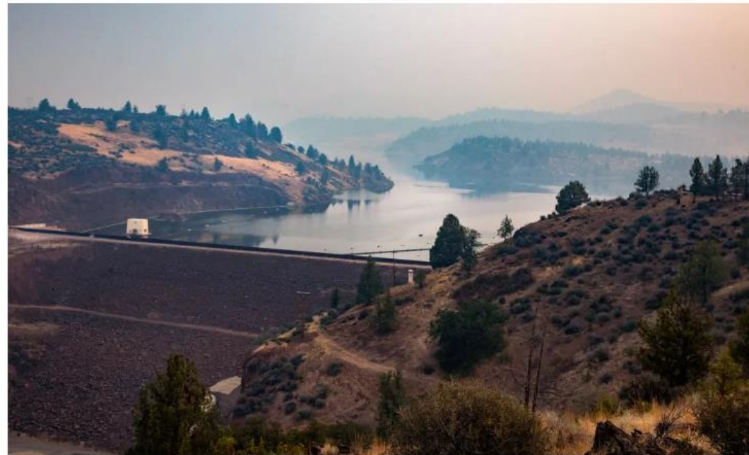
Iron Gate Dam in Hornbrook, California, on the Klamath River Brian van der Brue / Los Angeles Times via Getty Images
